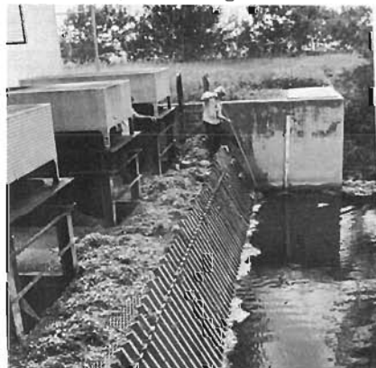
Fig. 2. Hygrophila polysperma clogging the pump intake screens of a drainage canal located in Coral Springs, Florida.
