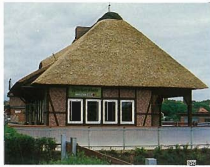
Figure 2. A building in Europe thatched with Common Reed (Photograph courtesy of David L. Sutton).
