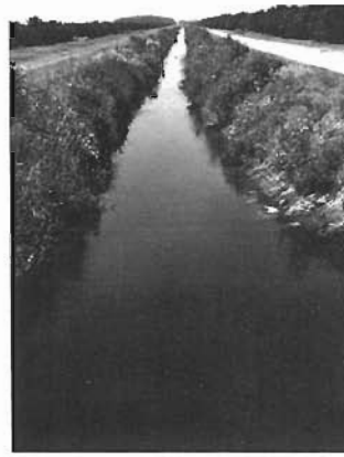
Figure 3: Canal free of aquatic weeds after use of mechanical methods and grass carp to manage plant growth.
