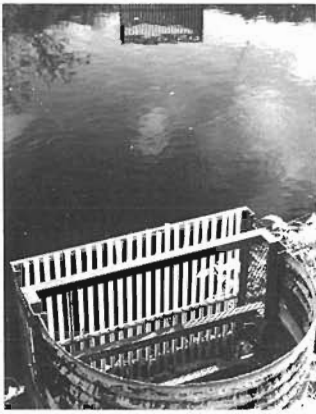
Figure 1: Fish barrier constructed of a single row of heavy gauge PVC (Polyvinylchloride) pipe to contain grass carp in agricultural waterways.
