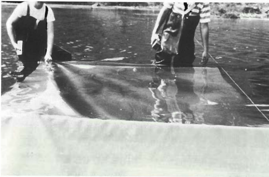
Fig. 4 Removable fiberglass screens, 7 by 100 feet, clear channels along shore and beside boat piers.
