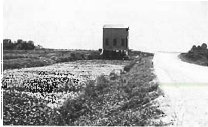
Water hyacinth clogging irrigation pump intake. File Photo.
