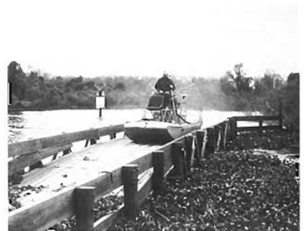
Wayne Corbin skids over airboat ramp used for passing over river dam. Photo by David Girardin.
