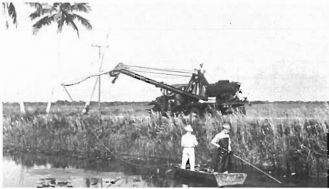
Hydrilla application, circa 1960, using a truck to pull the boat while a spray boom is held under the water for deep injection. Photo by Bob Blackburn.
