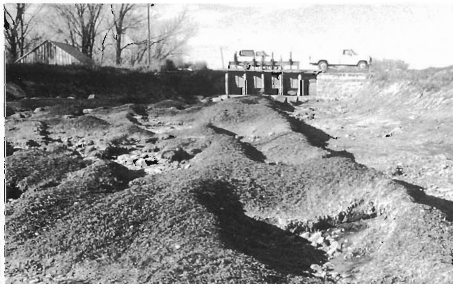
Figure 5. Silt deposition in a dewatered canal caused by the infestation of flowering-rush along the sides and across the bottom of the canal (silt has been removed from the right side of the canal to help meet water delivery requirements).
