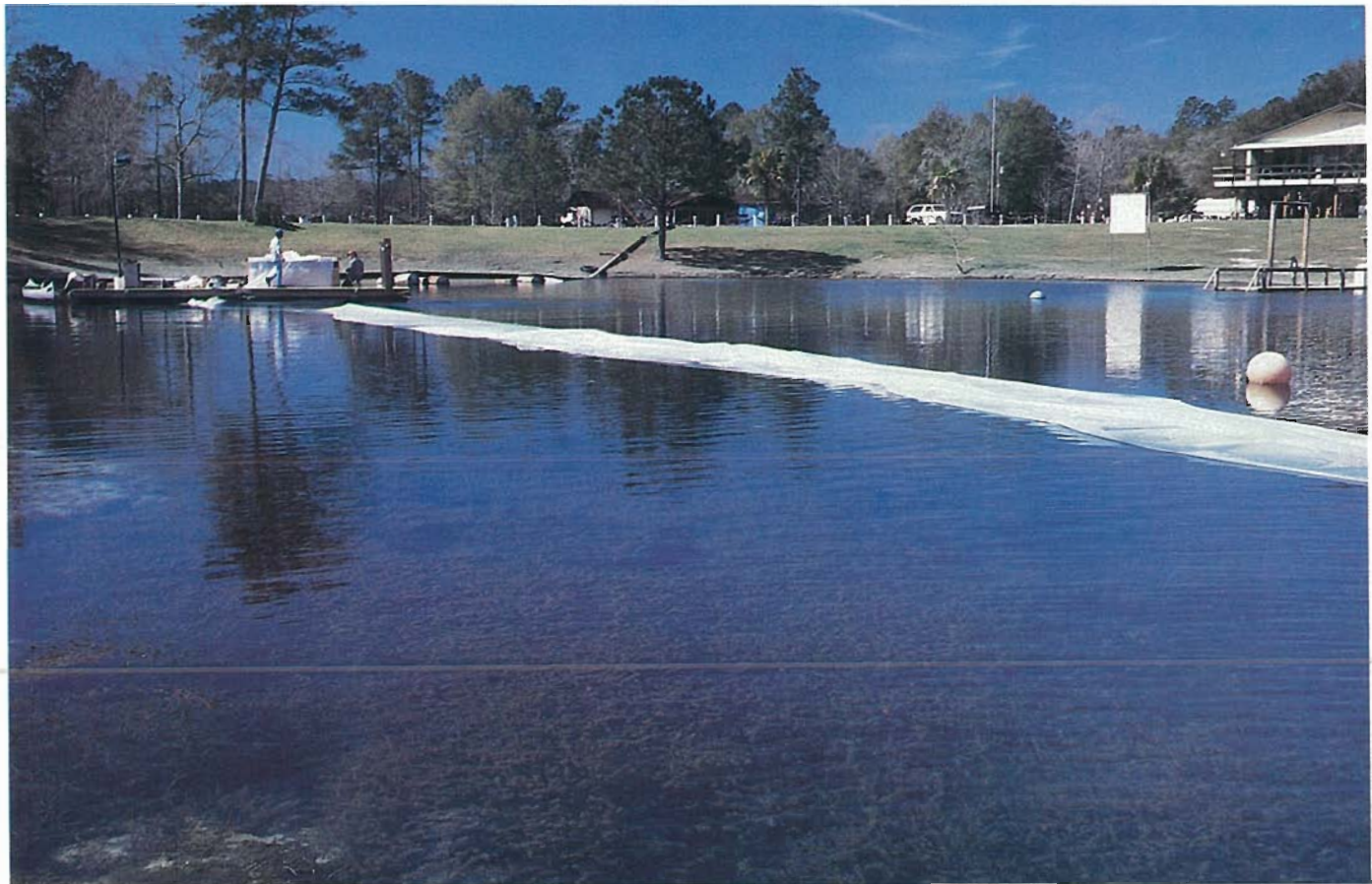
"Aqua control sleeve" being installed in Vortex Spring to divert the spring's flow 2,000 feet downstream. This allowed effective weed control in the main spring and spring run.
