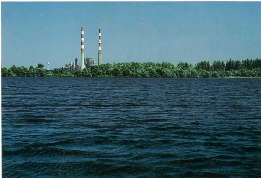
Portion of Sutton Lake looking toward power plant in June, 1992, two years after application of Sonar SRP.
