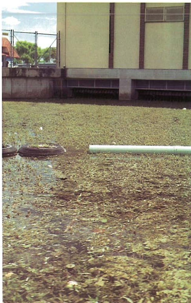
Figure 1. East Indian Hygrophila blocking water flow to a water control structure.
