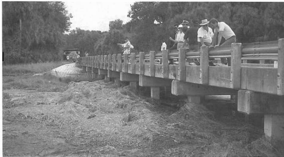
Figure 2. Floating mats of American frogbit and associated vegetation, such as this one, when allowed to reach large population levels in Upper Myakka Lake, have broken loose during high flows and required costly mechanical removal at bridges, by the Southwest Florida Water Management District.
