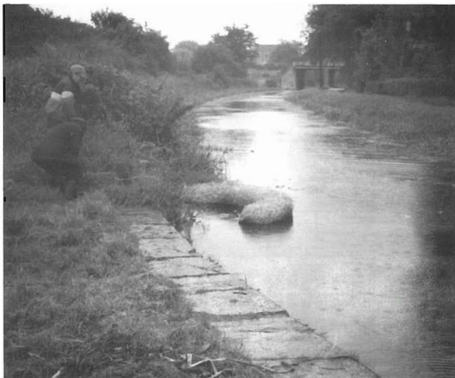
A barley straw "sausage" is applied for the purpose of controlling algae in a canal near Dublin, Ireland.
