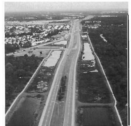
Figure 1. Aerial view of interconnected ponds along Kings Highway.
