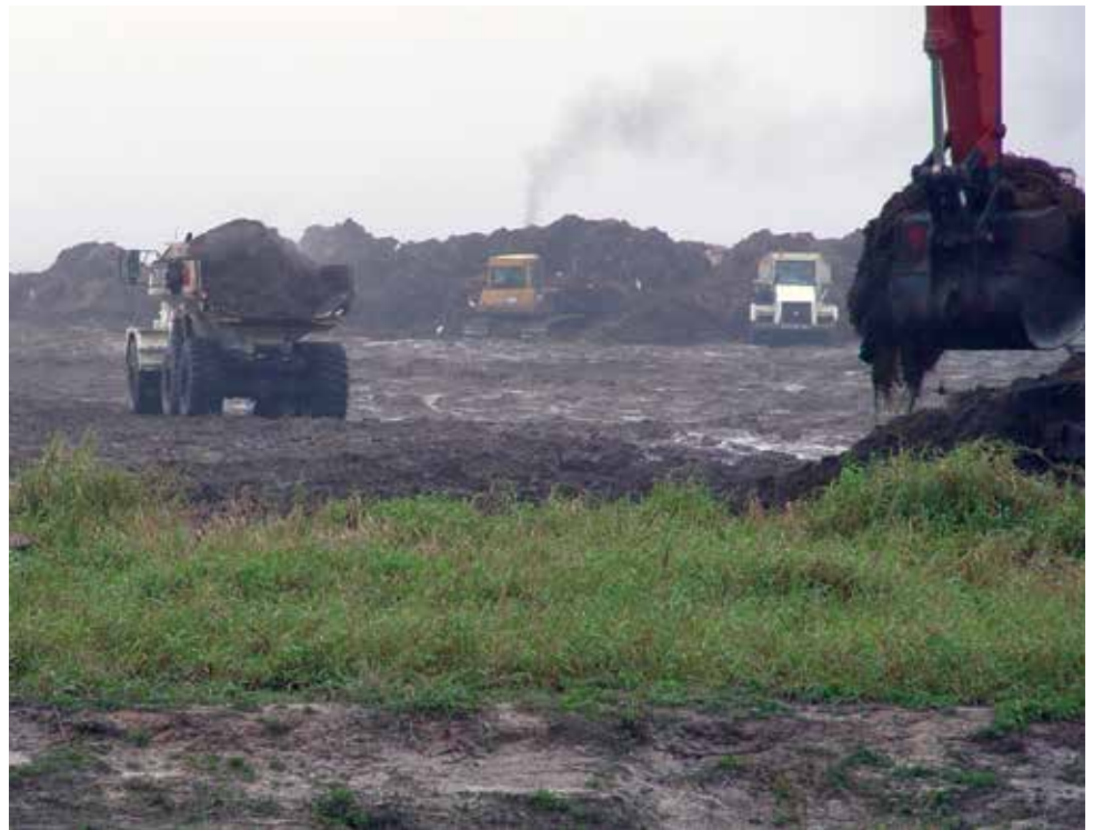
Figure 6. Muck removal and in-lake disposal creating islands of muck at Lake Tohopekaliga in 2003 (Credits: Mark Hoyer).
